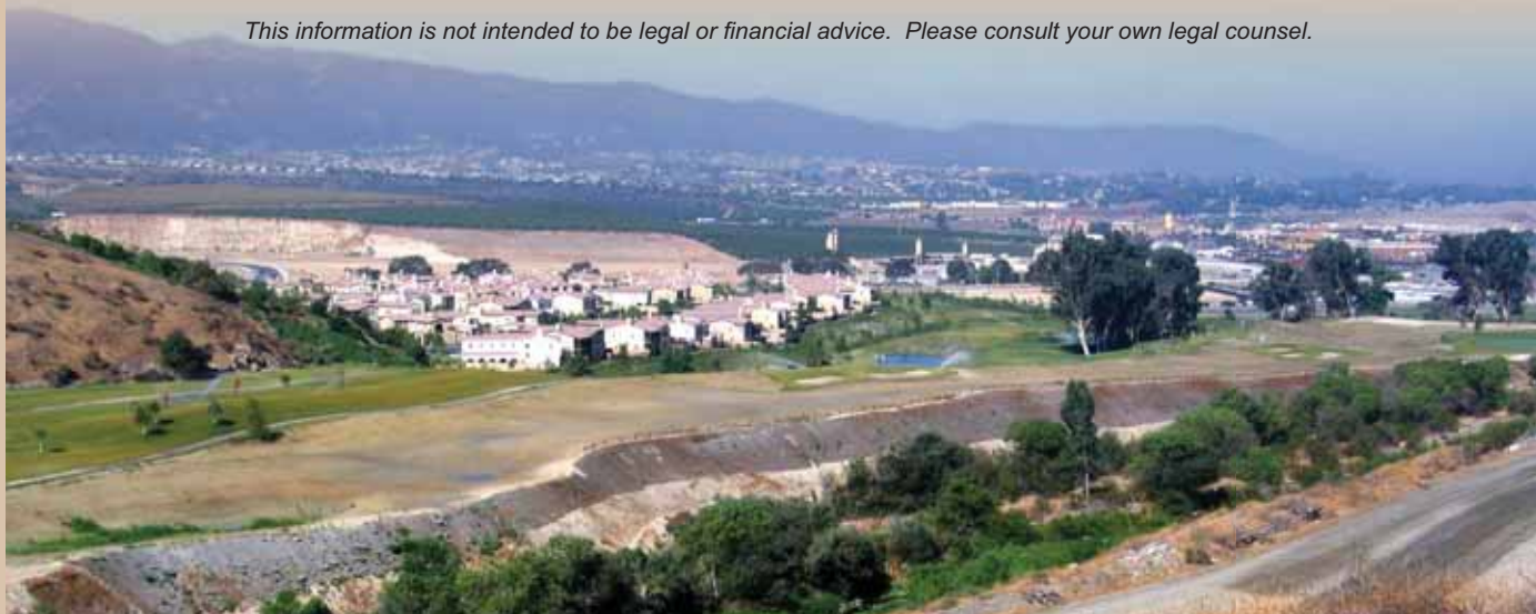
A wildlife corridor follows the Temescal Wash. Note the channel bank restoration and set-back of urban development.
