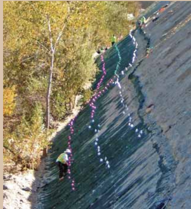
A woven, high performance mat was installed and interplanted with vegetation to strengthen the channel bank.
